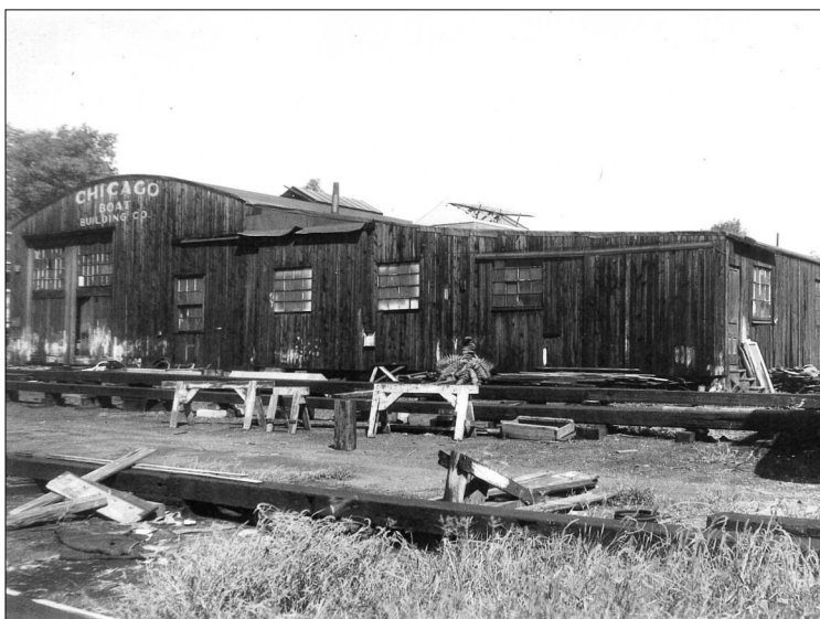
Greased 12x12 timbers were used as a rail system in the olden days to transport the boats through the yard. In the 50's the yard was paved and cradles were used.
