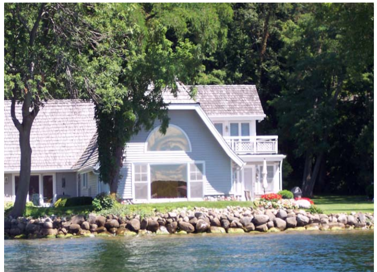
The boat house for HATHOR , with living quarters for the captain on the east side, was located on the western edge of the Ryerson property and still exists today as shown in this 2008 picture although the living quarters have been expanded and the launching ways from the boathouse to the lake have been covered over with grass and rocks which line the shore.
